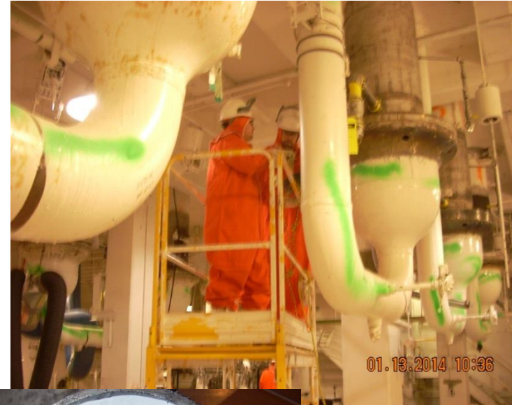
Removal of sodium-contaminated piping
